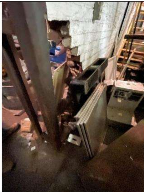
PHOTO 34 Location: Area 4/5 first floor Description: Significant portion of wall missing at opening
