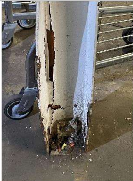
PHOTO 38 Location: Area 8 first floor Description: Typical damage to base of column.
