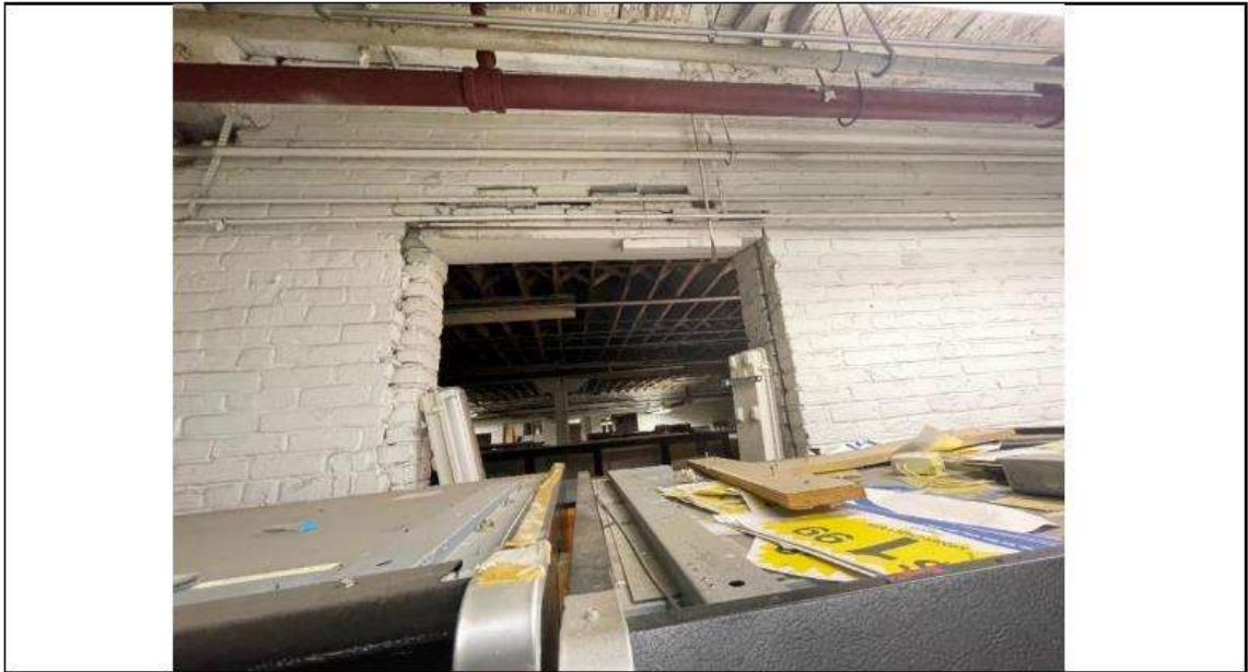
PHOTO 44 Location: Area 4/7 first floor Description: No header or lintel in this location
