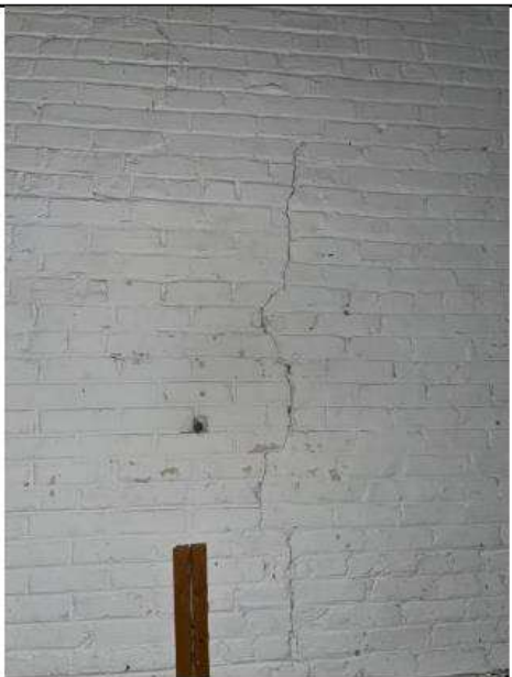
PHOTO 84 Location: Area 7 second floor Description: Crack in wall
