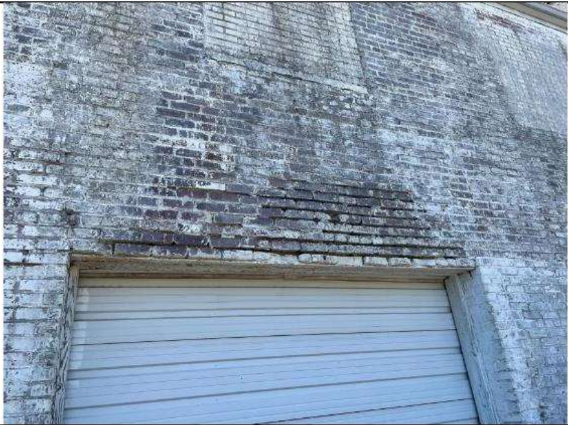
PHOTO 12 Location: Area 4 exterior Description: Voids in mortar and water staining
