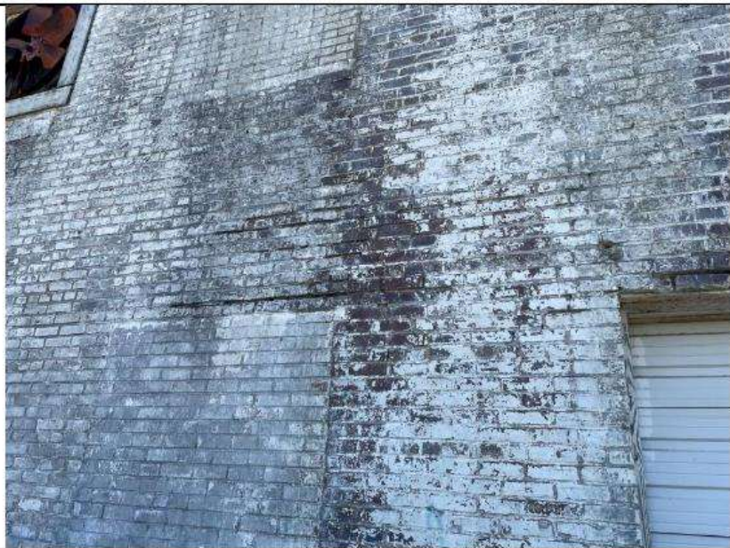
PHOTO 13 Location: Area 4 exterior Description: Voids in mortar and water staining
