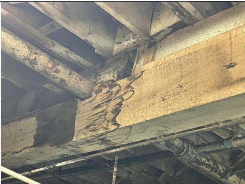
PHOTO 50 Location: Area 7 first floor Description: Staining on beam
