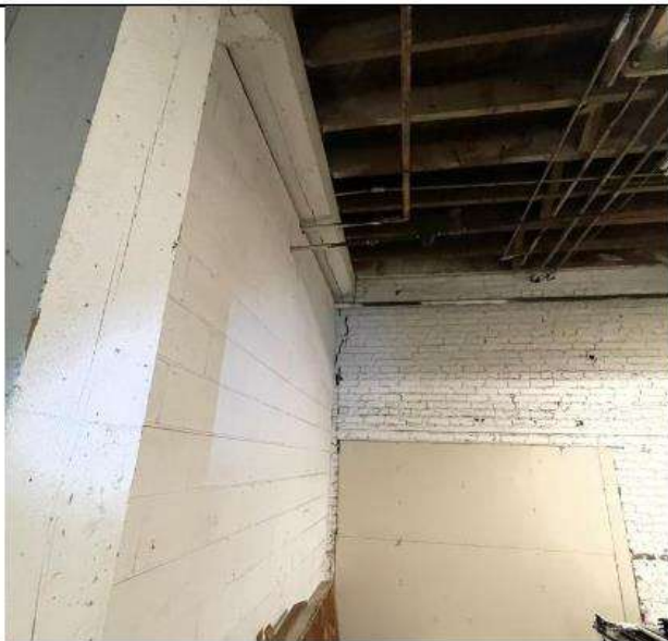
PHOTO 53 Location: Area 2 first floor Description: Significant damage to masonry at opening
