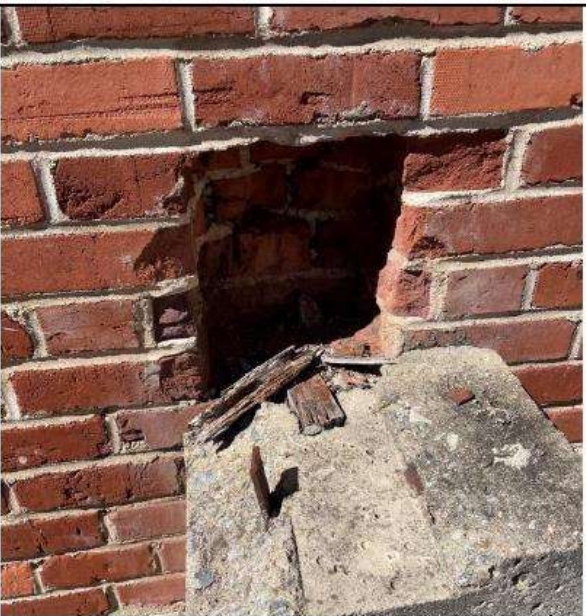
PHOTO 23 Location: Area 7 exterior Description: Holes in brick wall
