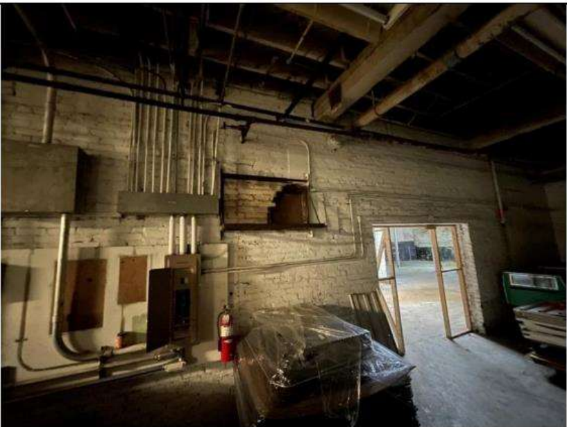
PHOTO 55 Location: Area 2 first floor Description: No header or lintel in this location
