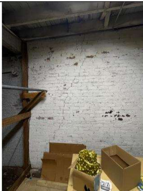
PHOTO 74 Location: Area 2 second floor Description: Crack in wall
