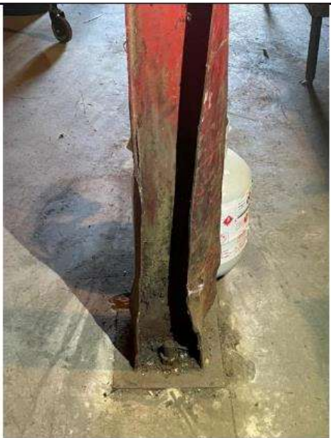
PHOTO 28 Location: Area 5 first floor Description: Damaged column
