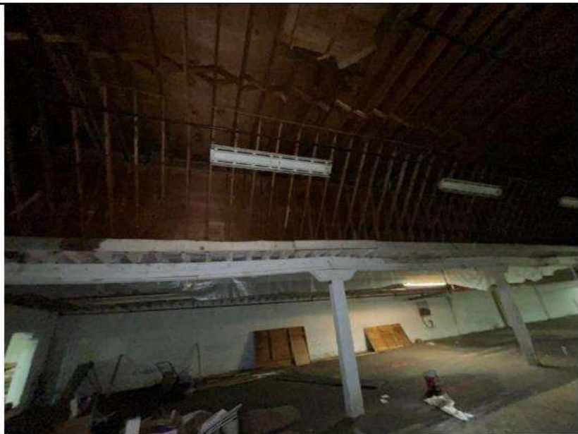
PHOTO 82 Location: Area 2 second floor Description: Sag in wood beam
