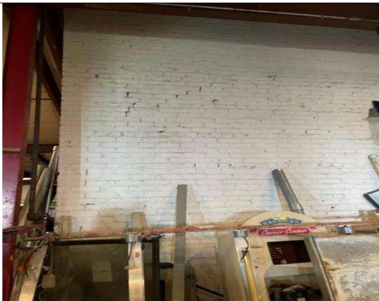
PHOTO 30 Location: Area 5 first floor Description: Cracks along wall
