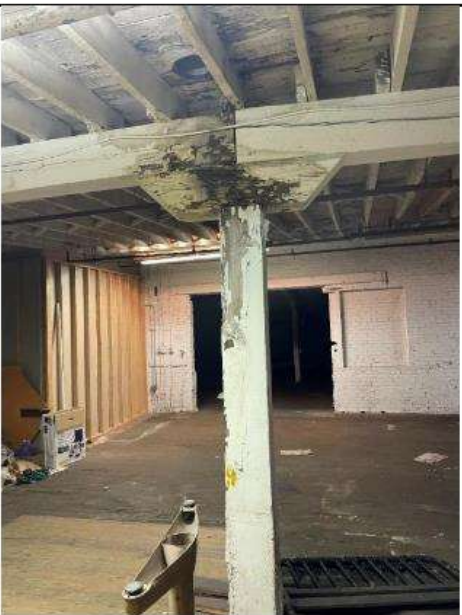
PHOTO 88 Location: Area 7 second floor Description: Water damage on column
