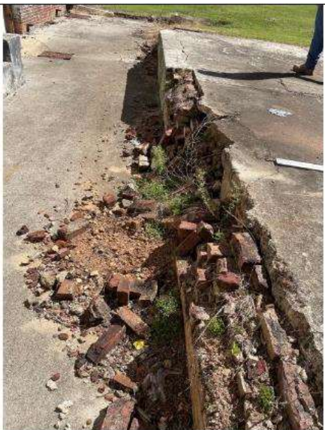
PHOTO 24 Location: Courtyard outside Area 7 Description: Damaged brick
