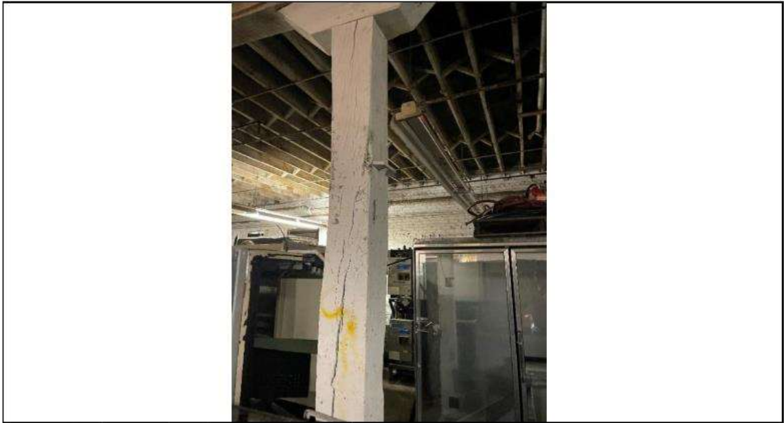
PHOTO 43 Location: Area 7 first floor Description: Crack in column
