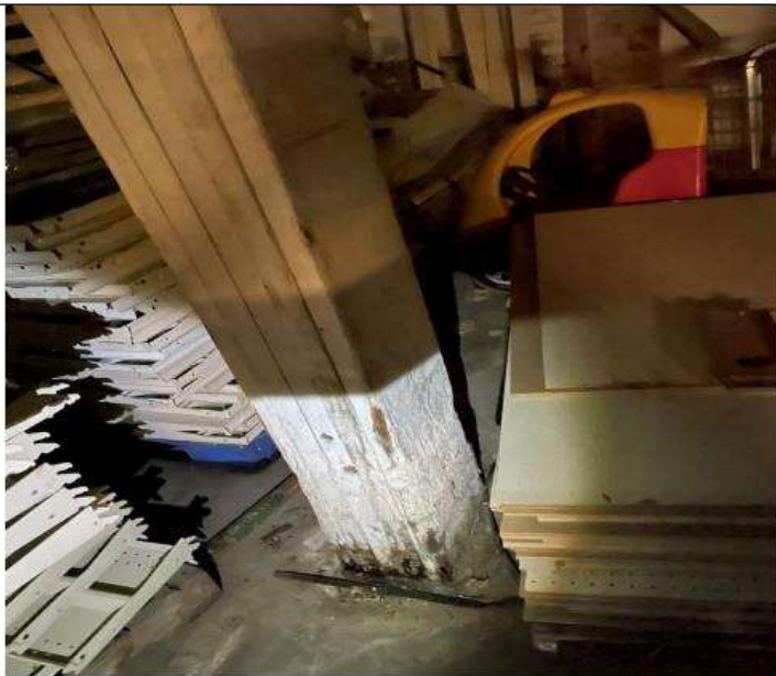
PHOTO 58 Location: Area 2 first floor Description: Column replaced by studs
