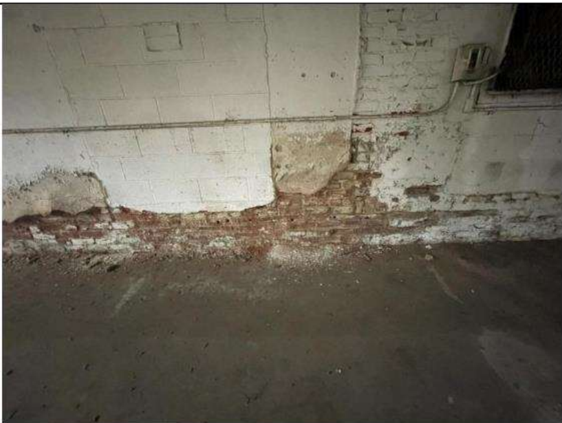
PHOTO 62 Location: Area 1 first floor Description: Soft/spalling brick
