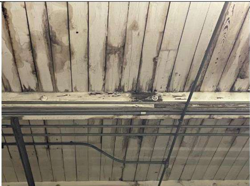
PHOTO 36 Location: Area 8 first floor Description: Water staining on framing above
