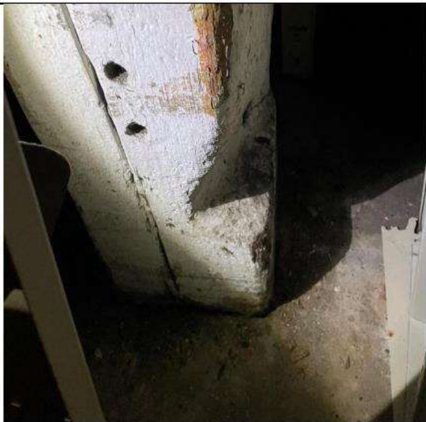
PHOTO 57 Location: Area 2 first floor Description: Crack in column
