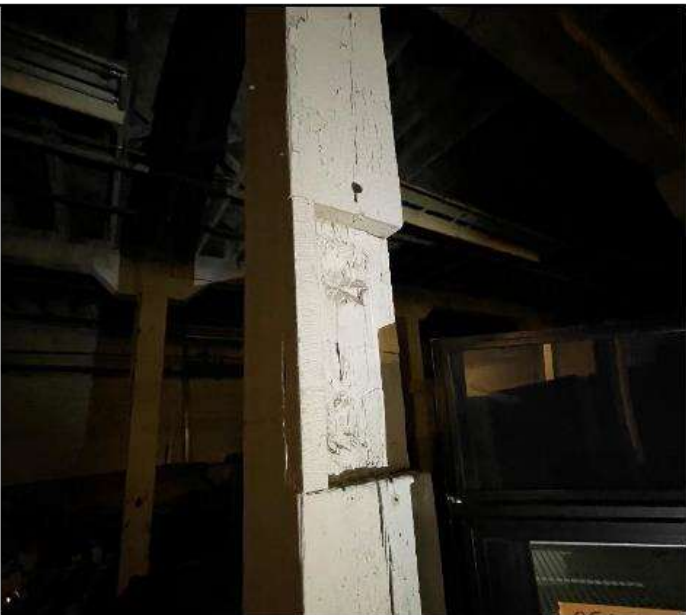
PHOTO 56 Location: Area 2 first floor Description: Crack in column and notch.
