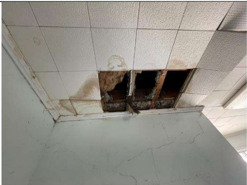
PHOTO 67 Location: Area 1 second floor Description: Water damage in ceiling
