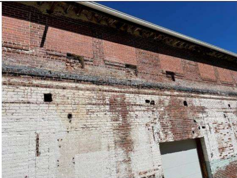
PHOTO 25 Location: Area 7 exterior Description: Cracking, holes in brick wall
