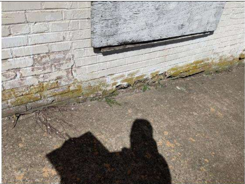
PHOTO 4 Location: Area 1 exterior Description: Minor mortar wash along base of wall at sidewalk
