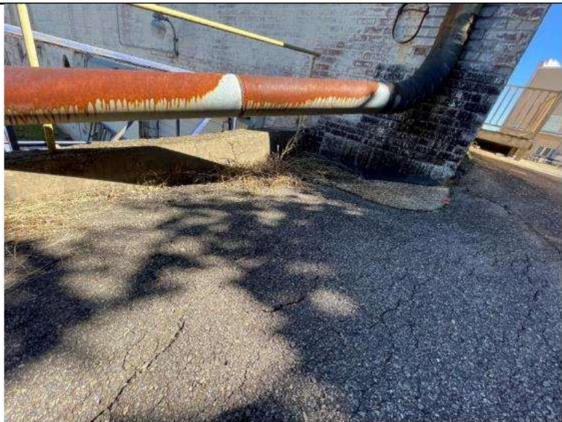
PHOTO 21 Location: Area 8 exterior Description: End of wall leaned inward. Ponding area.
