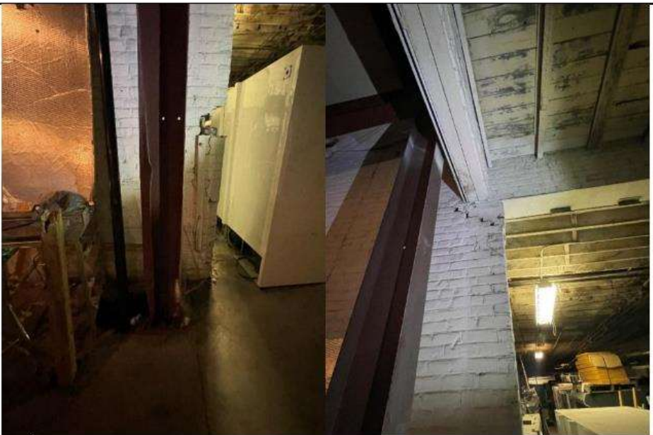
PHOTO 32 Location: Area 1/8 Description: Cracks in wall at bearing and damage below from an impact
