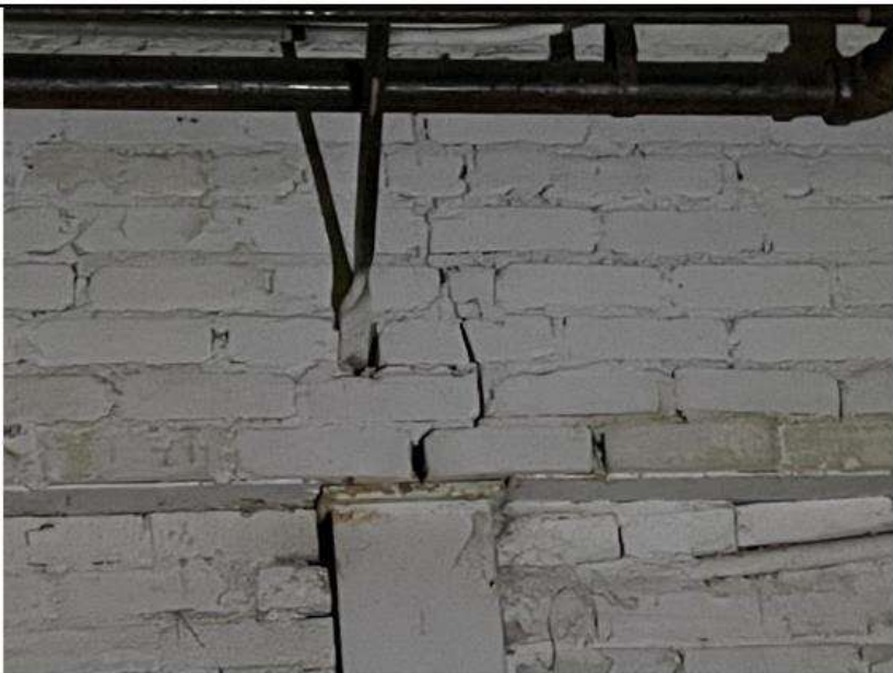
PHOTO 49 Location: Area 4 first floor Description: Crack in masonry above column
