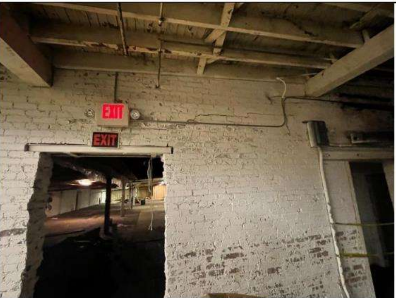
PHOTO 75 Location: Area 2 second floor Description: Cracks in wall around opening
