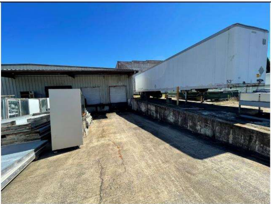
PHOTO 16 Location: Area 5 exterior Description: No railing on concrete wall. Wall has slight lean.
