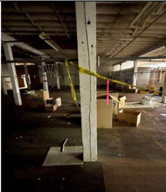
PHOTO 78 Location: Area 2 second floor Description: Crack in column
