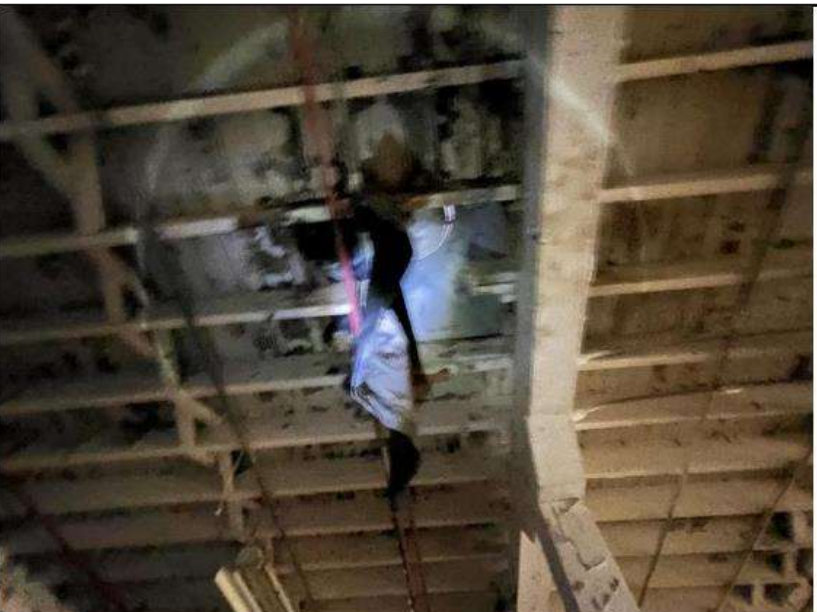
PHOTO 76 Location: Area 2 second floor Description: Rafter not properly blocked at exhaust
