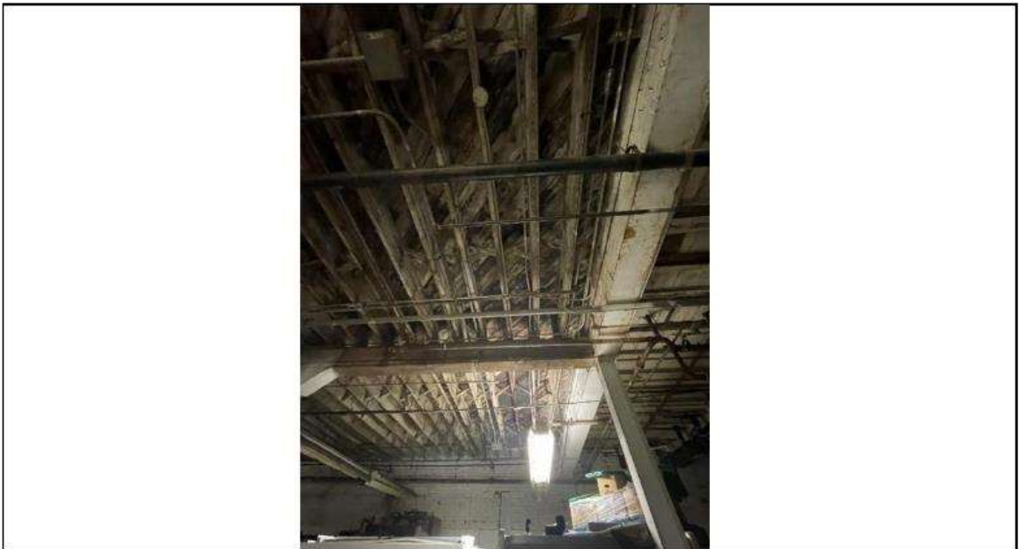
PHOTO 42 Location: Area 7 first floor Description: Water staining on framing above
