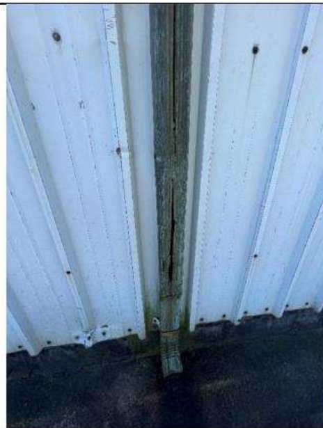
PHOTO 14 Location: Area 5 exterior Description: Split downspout
