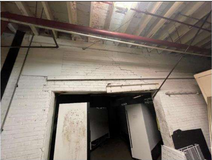
PHOTO 47 Location: Area 3/4 first floor Description: Severe cracking and deflection in header
