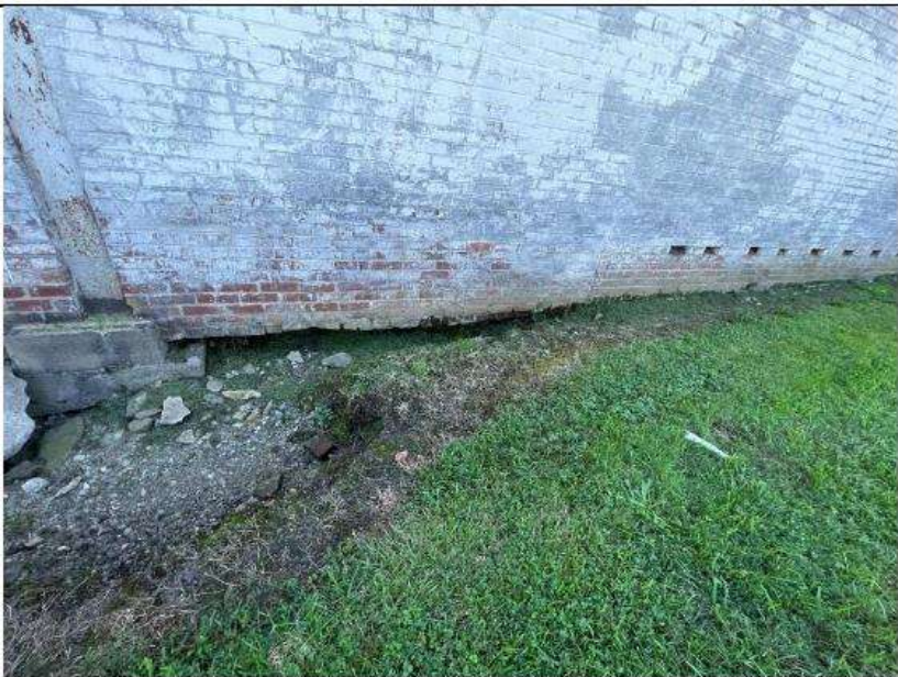
PHOTO 9 Location: Area 2 exterior Description: Undermining
