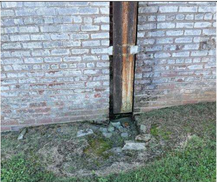
PHOTO 11 Location: Area 4 exterior Description: Drain exhibiting damage. Drainage to underdrain clogged.
