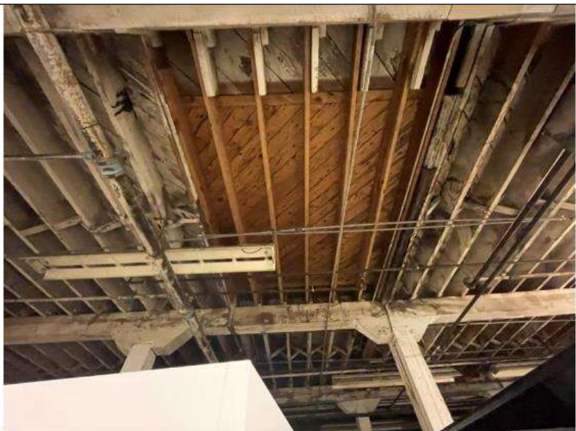
PHOTO 52 Location: Area 2 first floor Description: Infill in framing above
