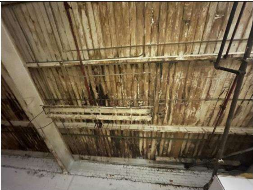
PHOTO 37 Location: Area 8 first floor Description: Water staining on framing above
