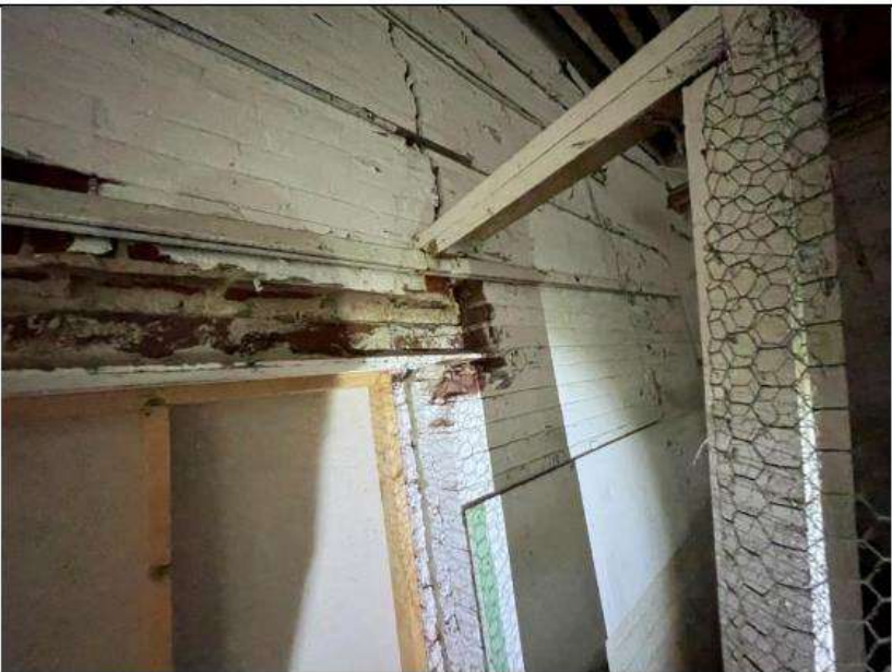
PHOTO 59 Location: Area 1 first floor Description: Significant damage to masonry at opening
