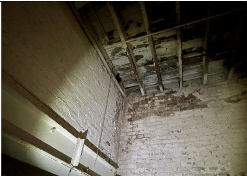
PHOTO 77 Location: Area 2 second floor Description: Water damage/staining roof and wall.
