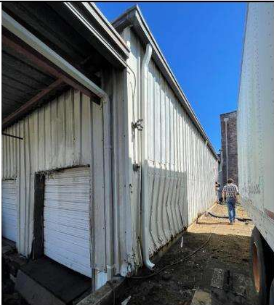
PHOTO 18 Location: Area 5 exterior Description: Damaged siding
