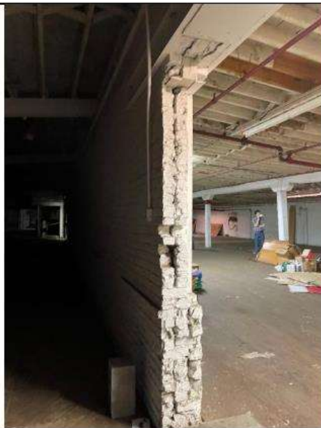
PHOTO 86 Location: Area 4 second floor Description: Rough cut opening
