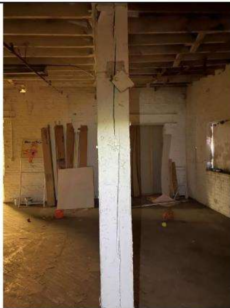
PHOTO 85 Location: Area 4 second floor Description: Cracked column
