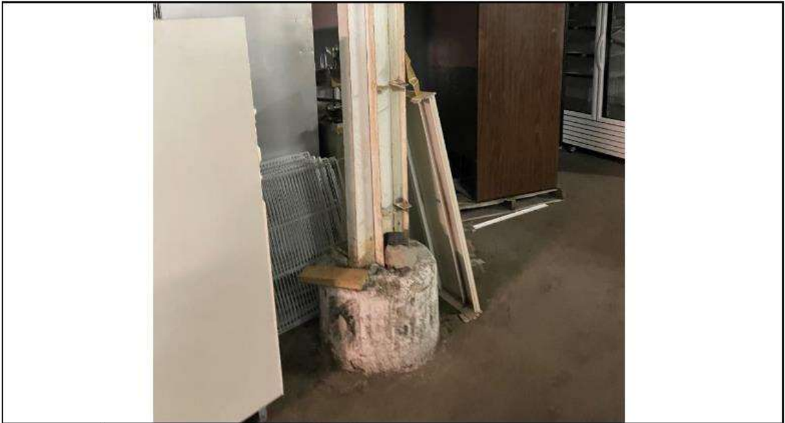
PHOTO 41 Location: Area 6 first floor Description: No anchor bolts attaching the column to the pier
