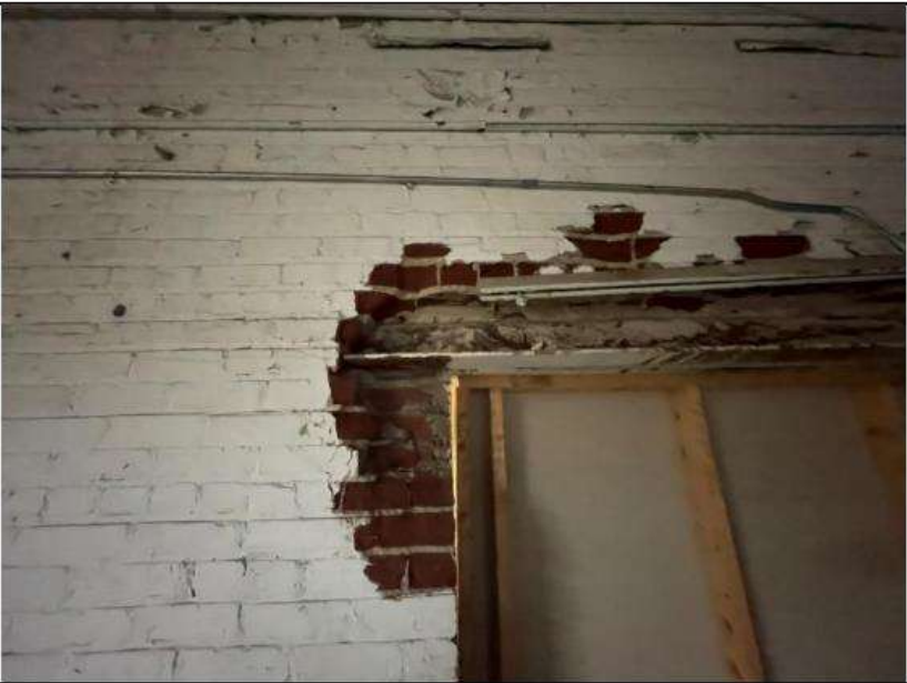
PHOTO 60 Location: Area 1 first floor Description: Significant damage to masonry at opening
