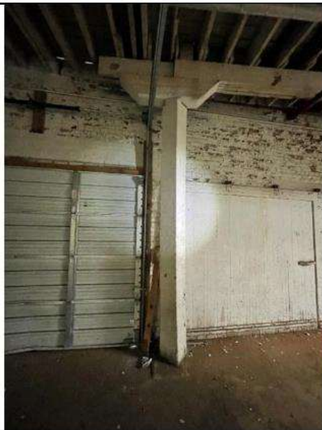
PHOTO 61 Location: Area 1 first floor Description: Column damaged, rotated
