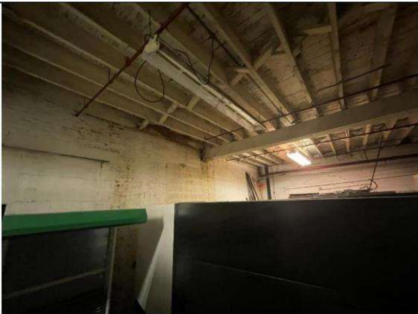
PHOTO 46 Location: Area 4 first floor Description: Stains in edge joist
