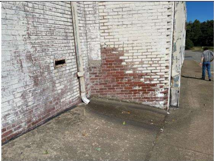
PHOTO 3 Location: Area 1 exterior Description: General condition. Minor wash around downspout and sidewalk
