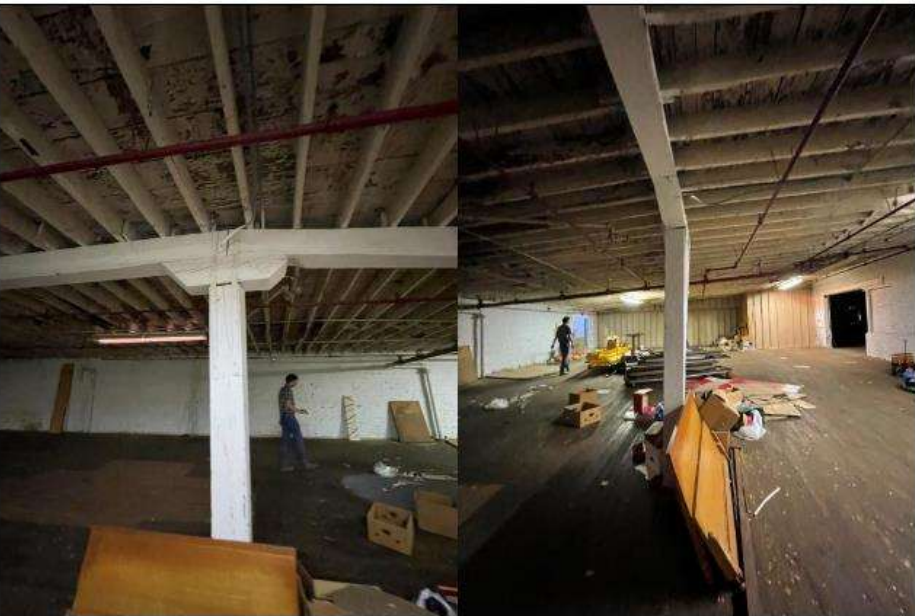
PHOTO 87 Location: Area 7 second floor Description: Column cracked and leaning
