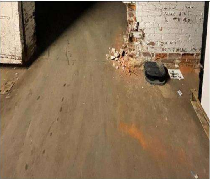
PHOTO 51 Location: Area 2/7 first floor Description: Soft brick at base of opening
