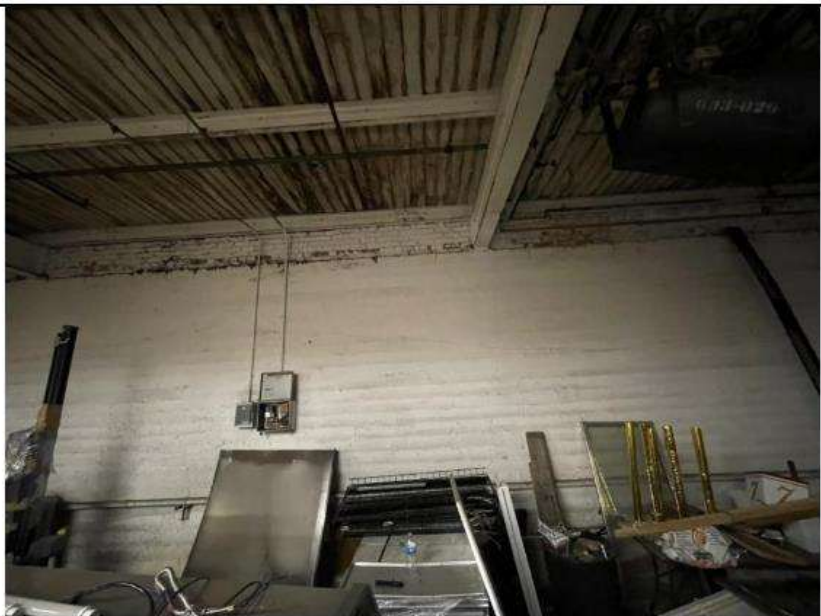
PHOTO 35 Location: Area 8 first floor Description: Water staining on framing above
