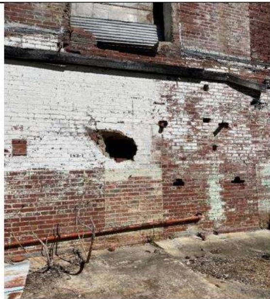
PHOTO 26 Location: Area 7 exterior Description: Cracking, holes in brick wall
