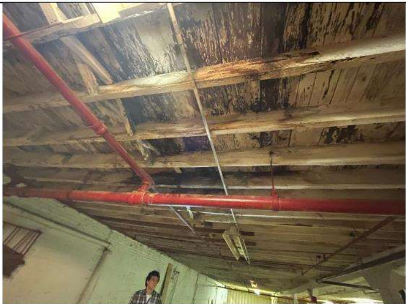
PHOTO 83 Location: Area 7 second floor Description: Water damage in ceiling
