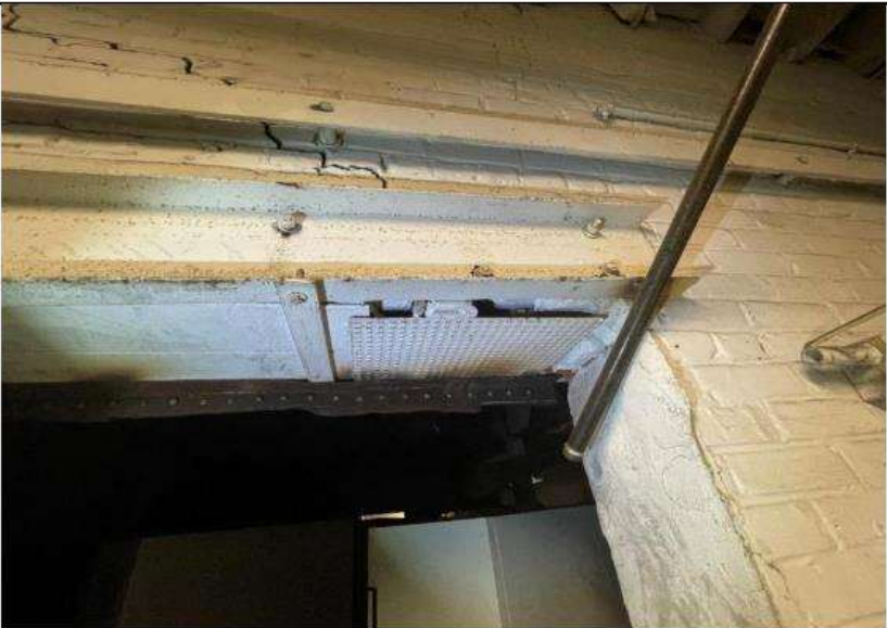
PHOTO 48 Location: Area 3/4 first floor Description: Severe cracking in header
