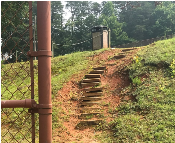
Safety concern – exposed rebar and no handrail on stairs at Chatham Heights Park
