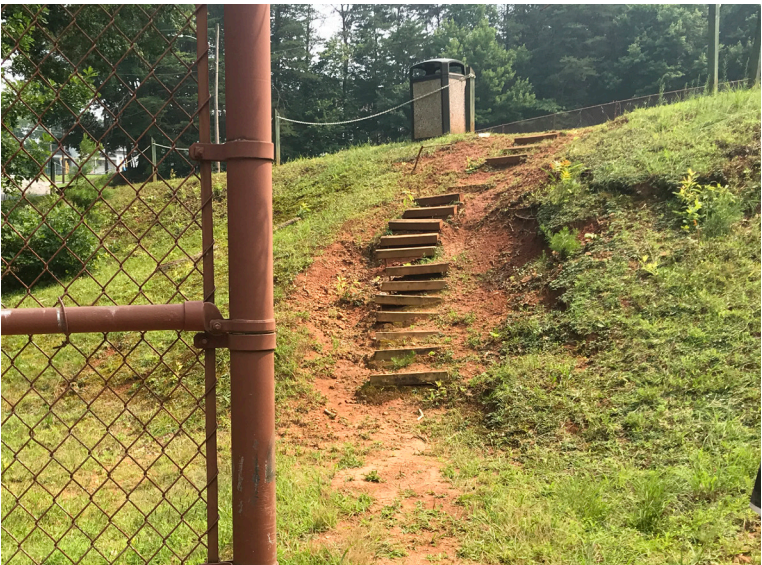
Safety Concern (1) - exposed rebar and no handrail on stairs at Chatham Heights Park
